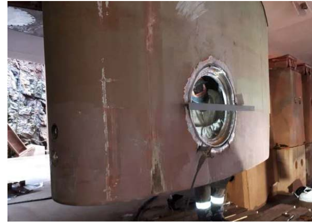
MS 70 installation at port drop keel
