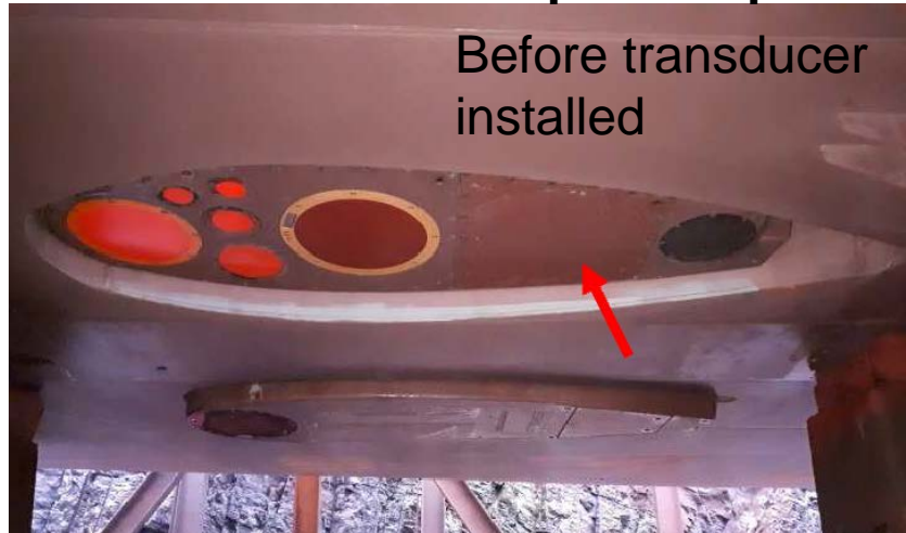
ME 70 installation at port drop keel
